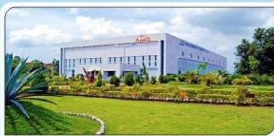
Works at Nagpur
