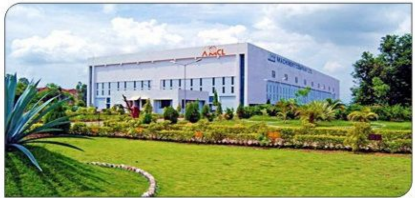
Works at Nagpur
