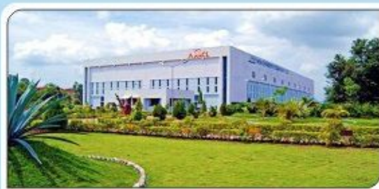
Works at Nagpur
